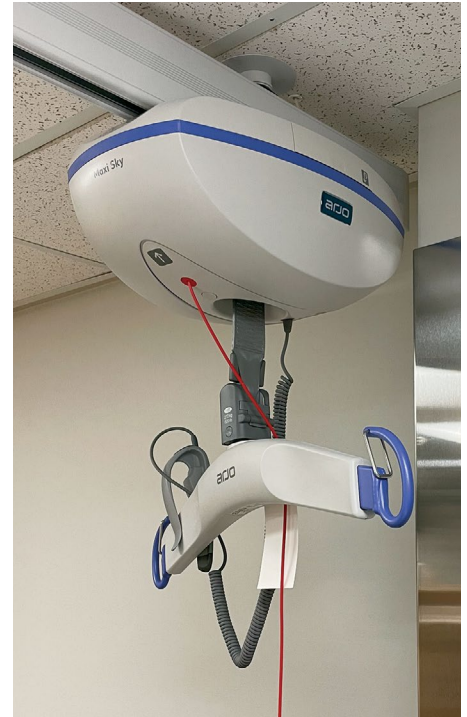
Newly installed ceiling mounted patient lift in the updated MRI suite.
